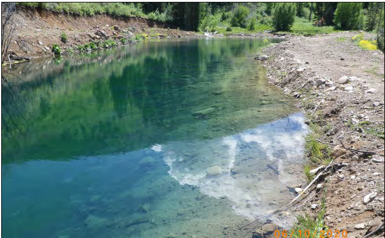
Constructed pond facing east. Davenport Creek is off the photo to the right of the earthen berm. The water source for the pond, inflow from off-site springs, is visible at top center of photo.
